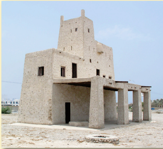
The tower from the north
